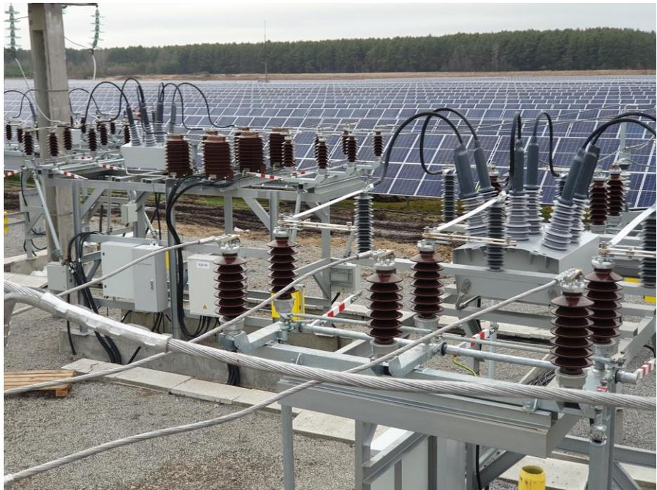
*NOJA Power OSM Reclosers used to connect a 17 MW Solar Farm to the Medium Voltage Distribution Grid.*
