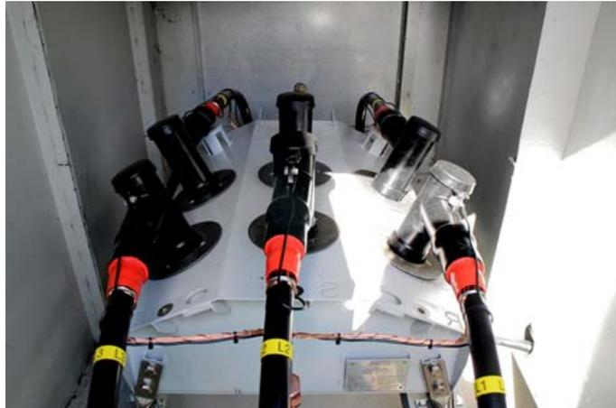
*OSM Recloser with DIN Profile Dead Break Elbow Connections in a Kiosk Installation*
