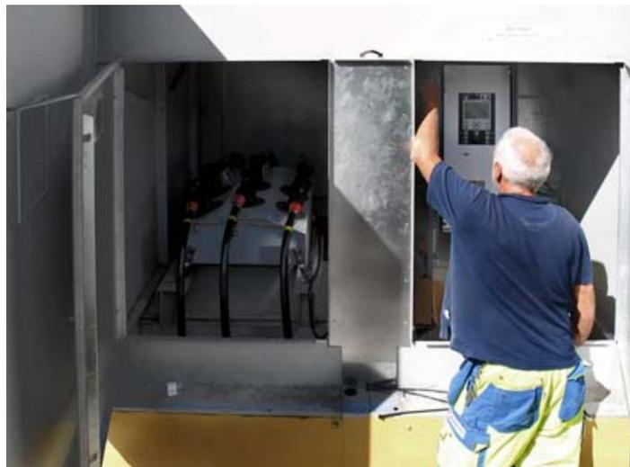
*OSM Recloser in an underground cable protection Kiosk in Sweden*
