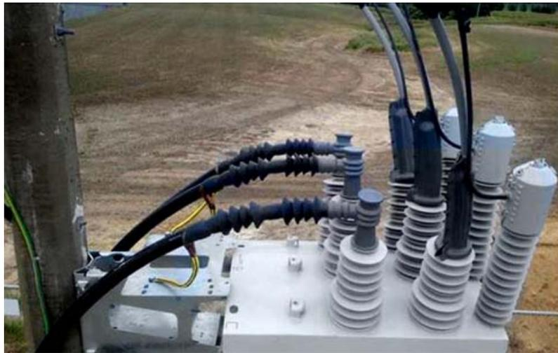
*NOJA Power 38kV OSM Recloser with Overhead and Underground Cable Terminations*
