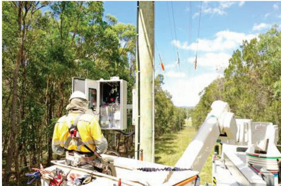
*The first NOJA Power RC20 Controller with PMU capability commissioned in service.*
