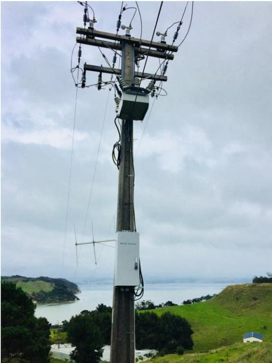
miraculous when observed in isolation. The RC10-200 upgrade path is a replacement of the control system, allowing utilities to maximise the return on investment in primary assets and essentially eliminating the High Voltage work required in a switchgear site upgrade.
