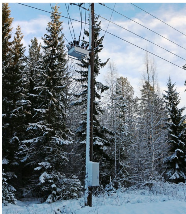
Typical installation design, OSM Recloser with RC Series Control
